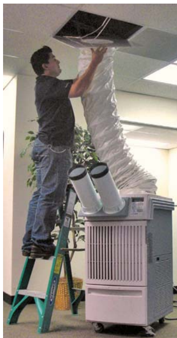
A technician installs a portable-cooling exhaust kit.
